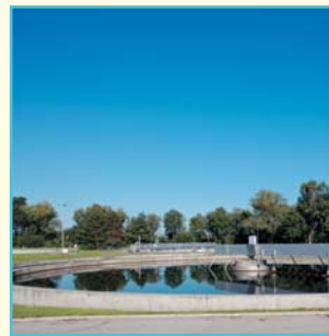
The treatment of mixed water in purification basins has been used at the treatment plant in Wulkaprodersdorf for decades.
