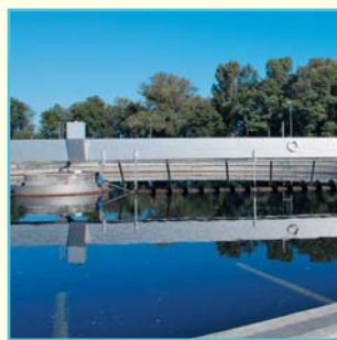
The method of mixed water treatment in purification basins helps the treatment plants to save money.
